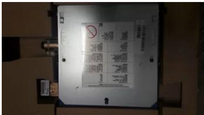
TAC20602A995 Overspeed governor LH V_n=1.75 m/s, V_p=2.21 m/s OTIS
